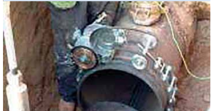
22" Water main being cut with the Keel Cutter
